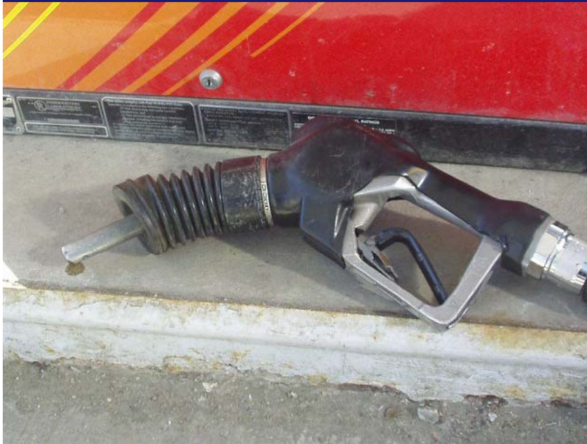
Vapor Balance System Stage II Vapor Recovery
